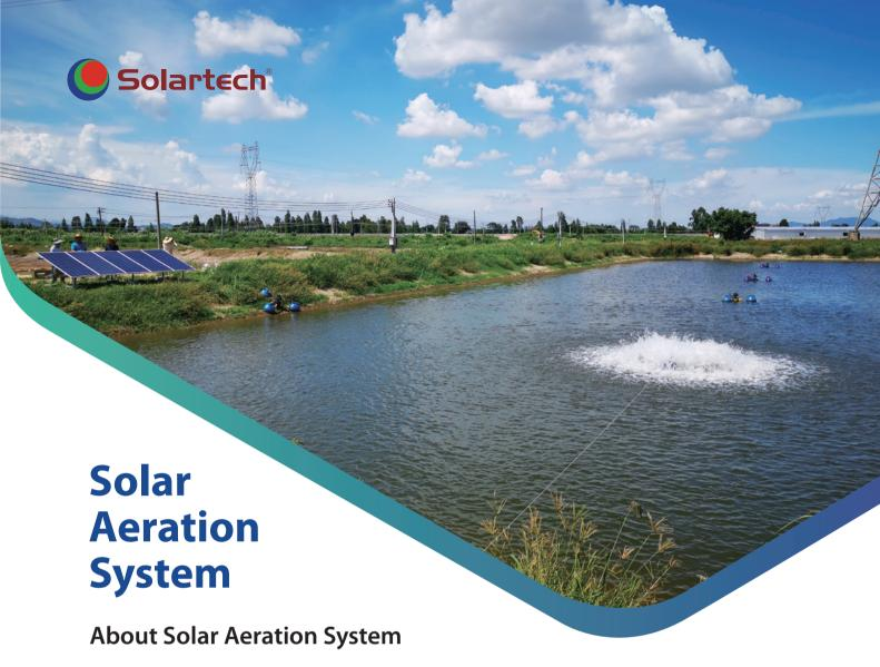
It is developed for the application scenarios of fish pond oxygenation for fish farming. The system mainly consists of solar arrays, solar inverters and aeration pumps.
