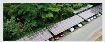
1,000m2 solar car parking lot, using amorphous silicon thin film solar panels, grid connected power generation, which is used for landscape lighting and electric vehicle charging;
