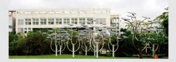
solar tree, using polycrystalline silicon solar panels, grid connected power generation to provide power for landscape lighting and fountains.
